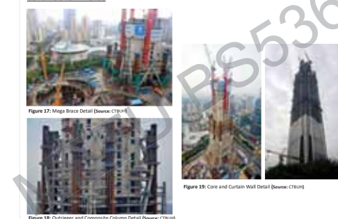
Figure 17: Mega Brace Detail (Source: CTBUH) Figure 18: Outrigger and Composite Column Detail (Source: CTBUH)
